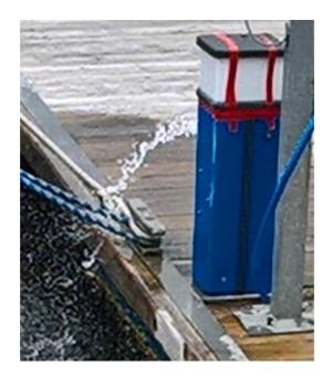
The resulting fountain meant that water pressure was dropping all over the marina. As the harbour master from the Tobermory Harbour Association disappeared to shut off the supply I deployed a wooden bung normally used to fix boat leaks. I tapped it into the remains of the fitting to block the outflow and hence service was restored to the rest of the marina.
